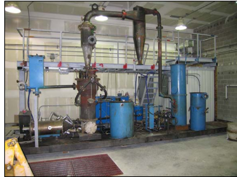
Test rig at Saskatchewan Research Council, Canada
